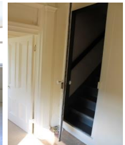
Walk in attic (storage)
